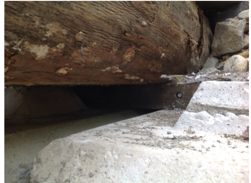
left bank sill
