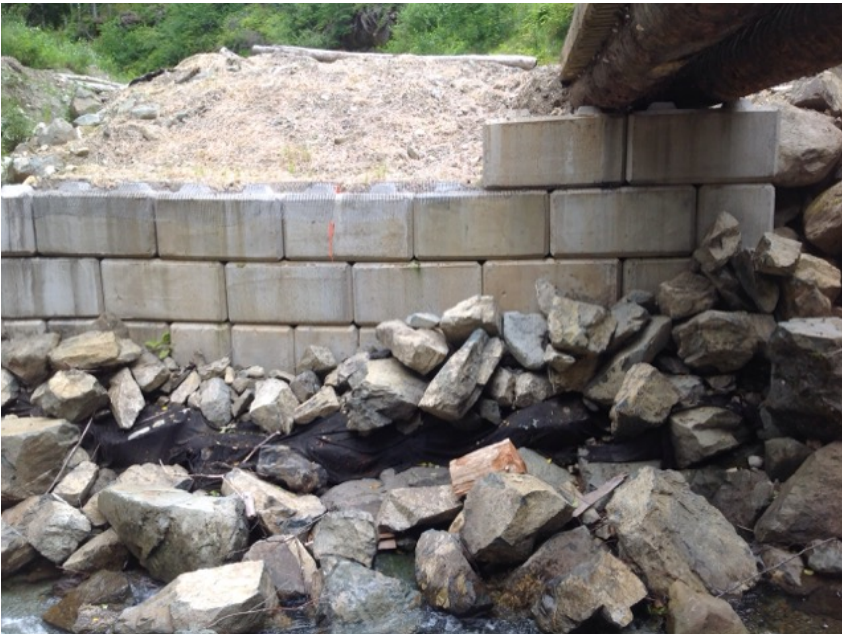
Right Bank Abutment when facing downstream
