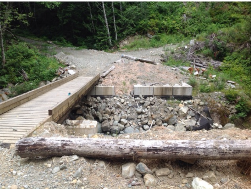
Approach from Right Bank when facing downstream
