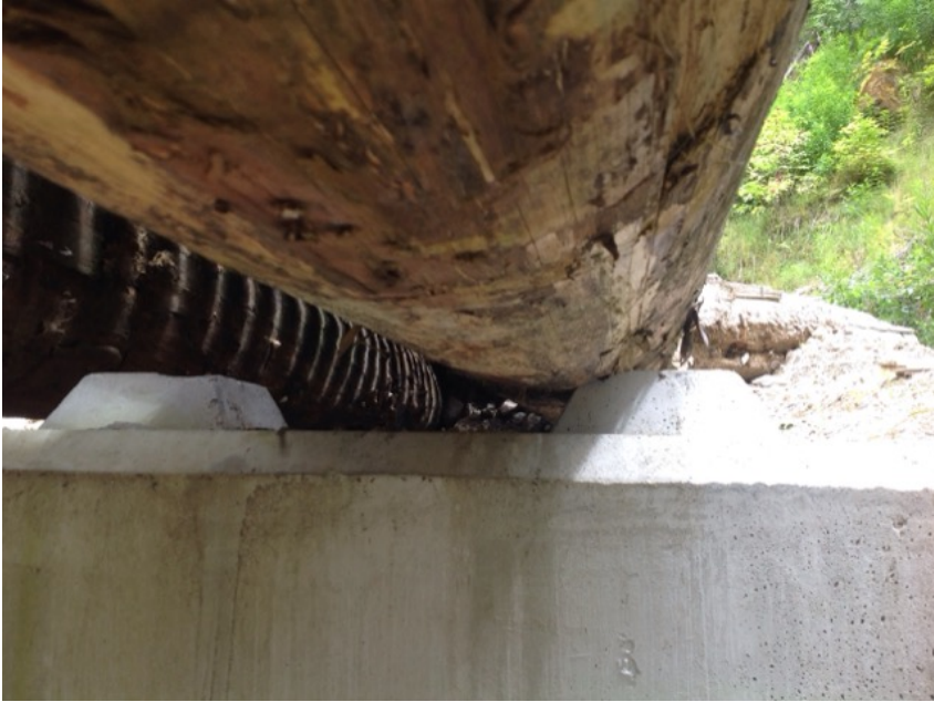
partial bearing on right bank
